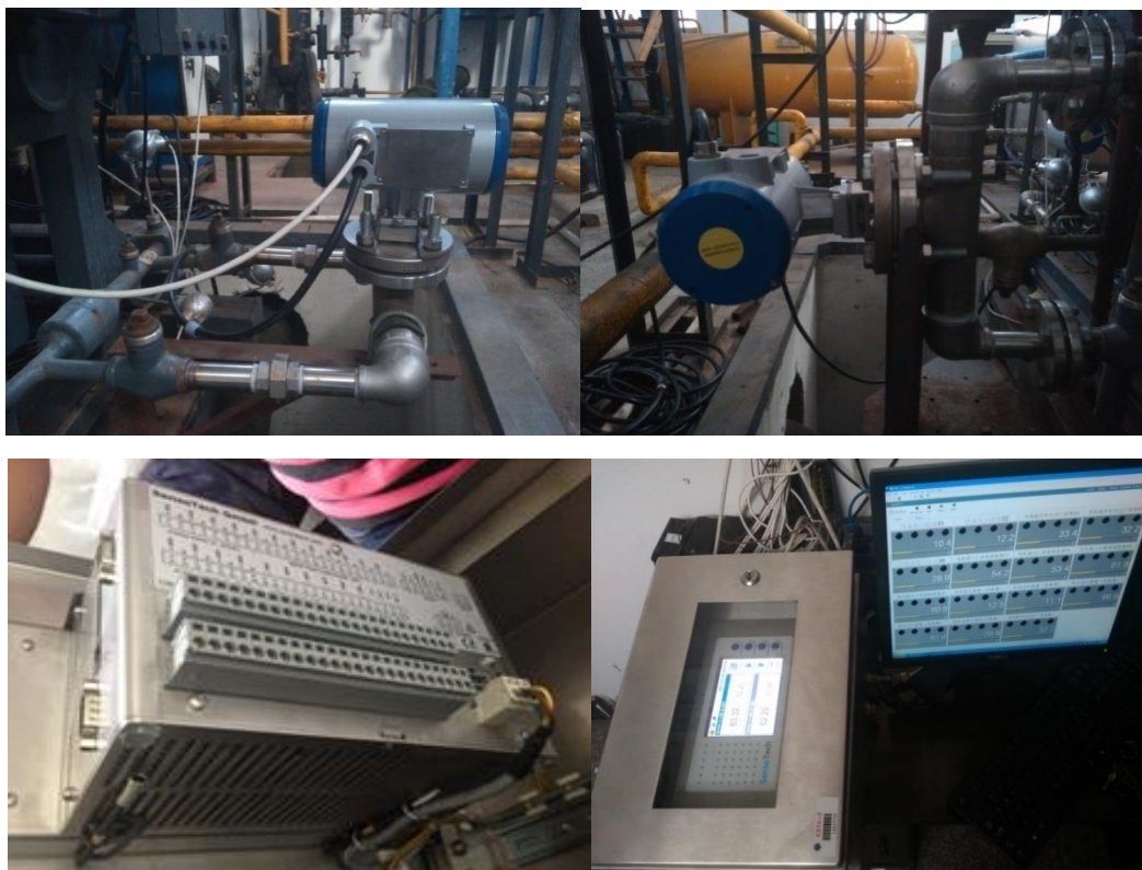
Figure 4-3. Photos of the in-line ultrasonic concentration sensor.
